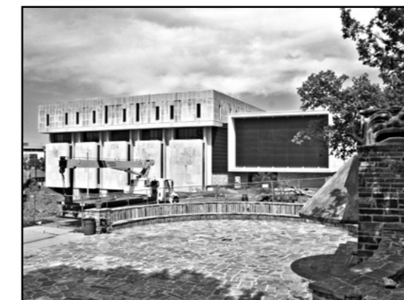
Construction begins on the Miller Nichols Library expansion behind the University Playhouse.
