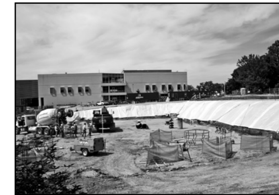
JE Dunn workers begin construction on the Henry W. Bloch Executive Hall for Entrepreneurship and Innovation.
