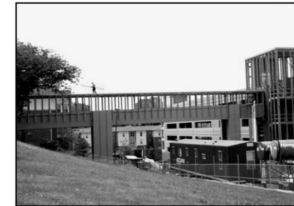
Skywalk from the Cherry Street garage to the Student Union.
